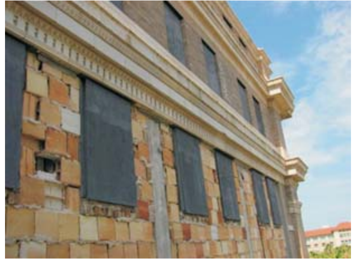
Image 5. Hollow clay tile & brick infill
