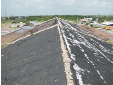
Image 6. Current Roof Condition
